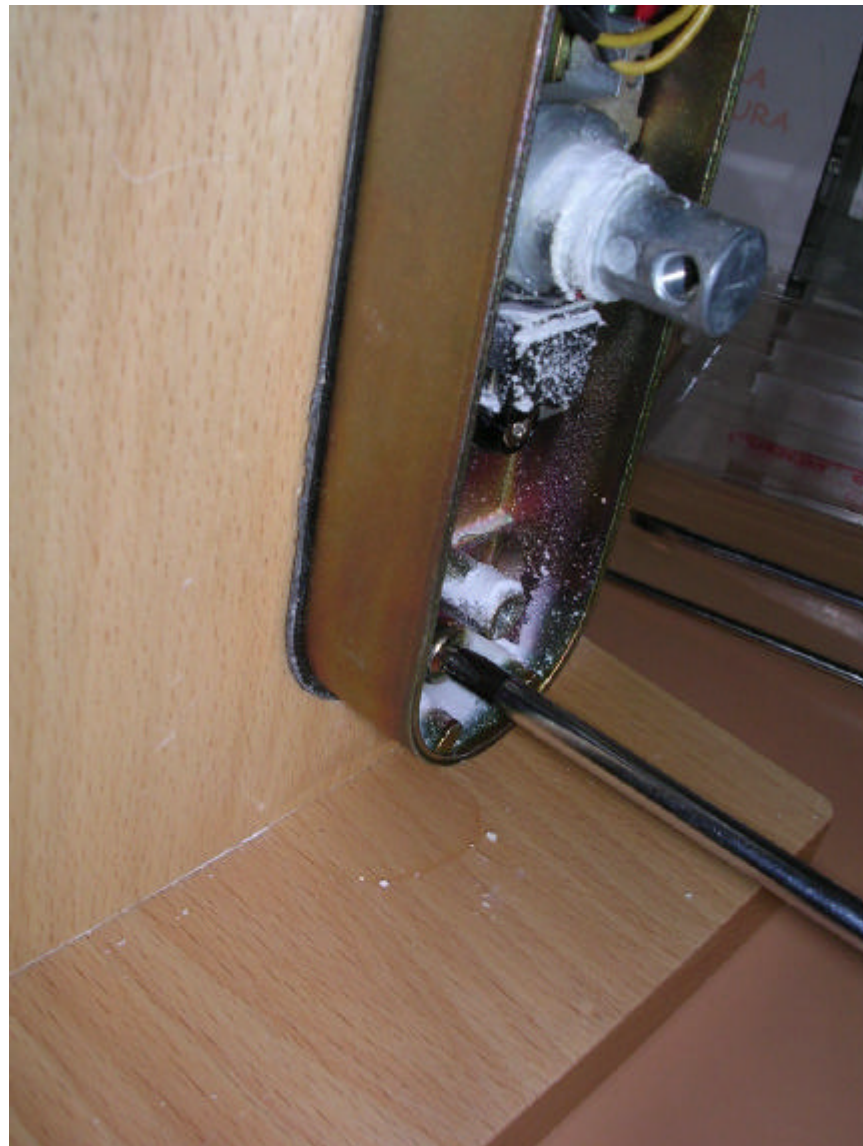
Inside the equipment under test (at the bottom), ingress of water.
